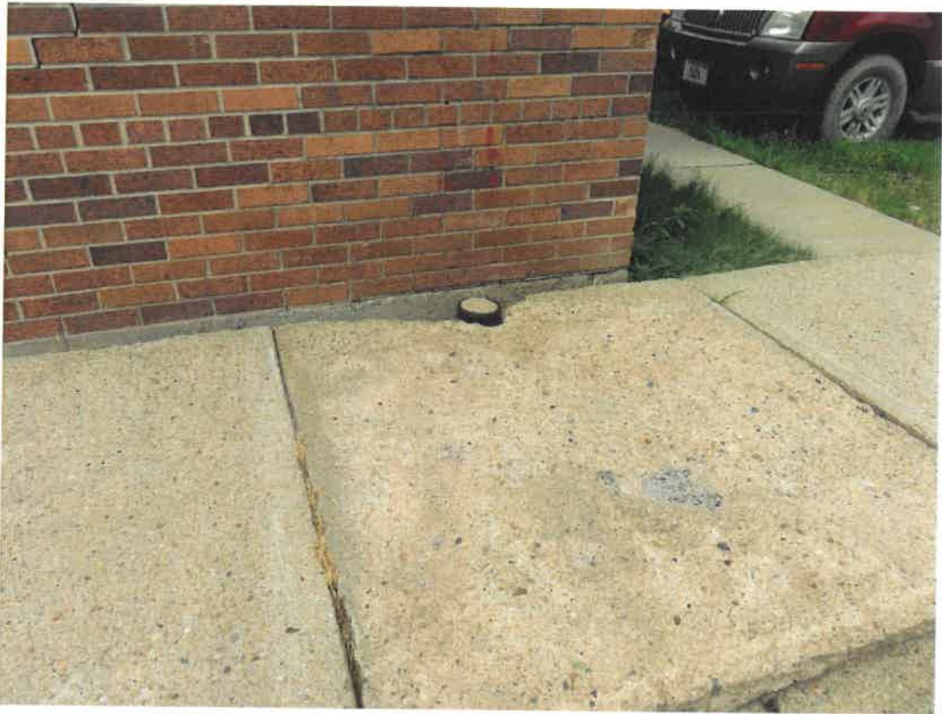
Photo 25 – Typical Drainage Issue on East Wall w/ Missing Downspout, Capped Drain Line and Severely Corroded Sidewalk
