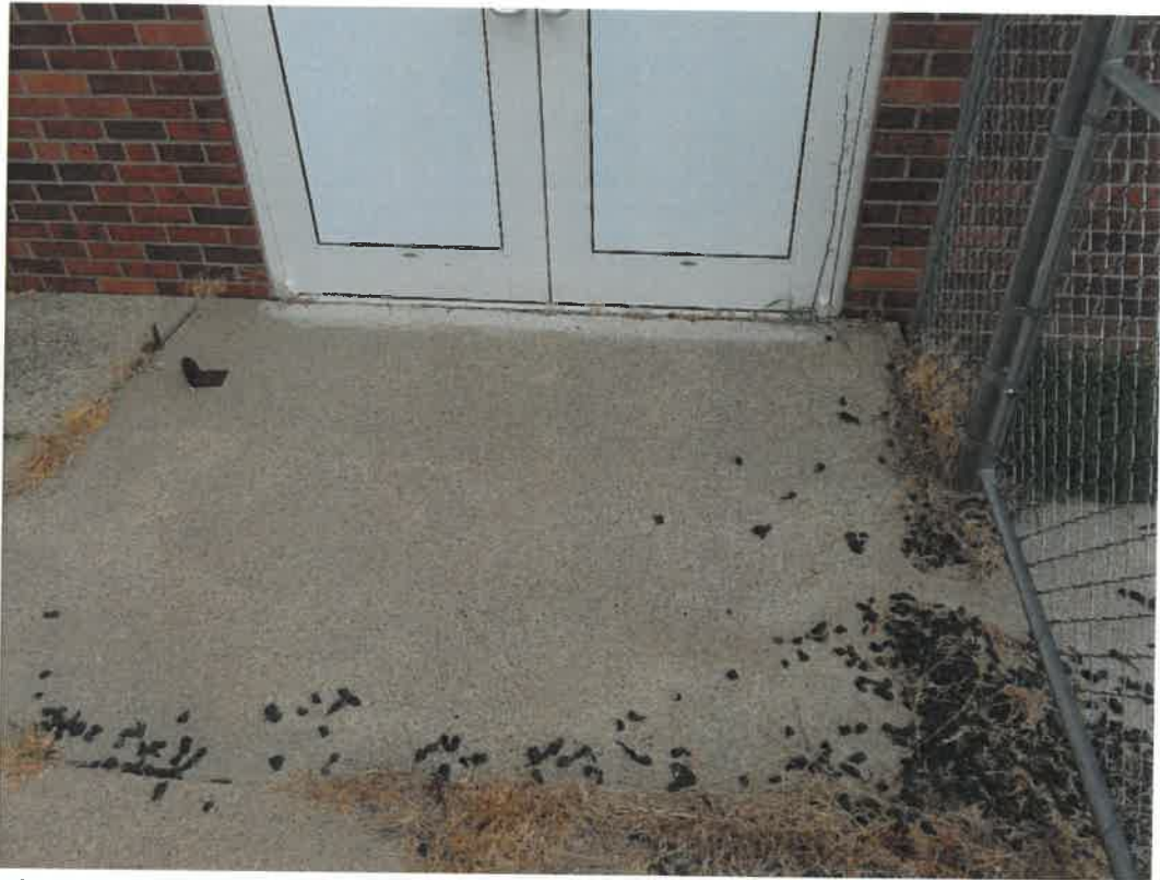
Photo 27 – Low Spot in Sidewalk at Walk Door in West Wall
