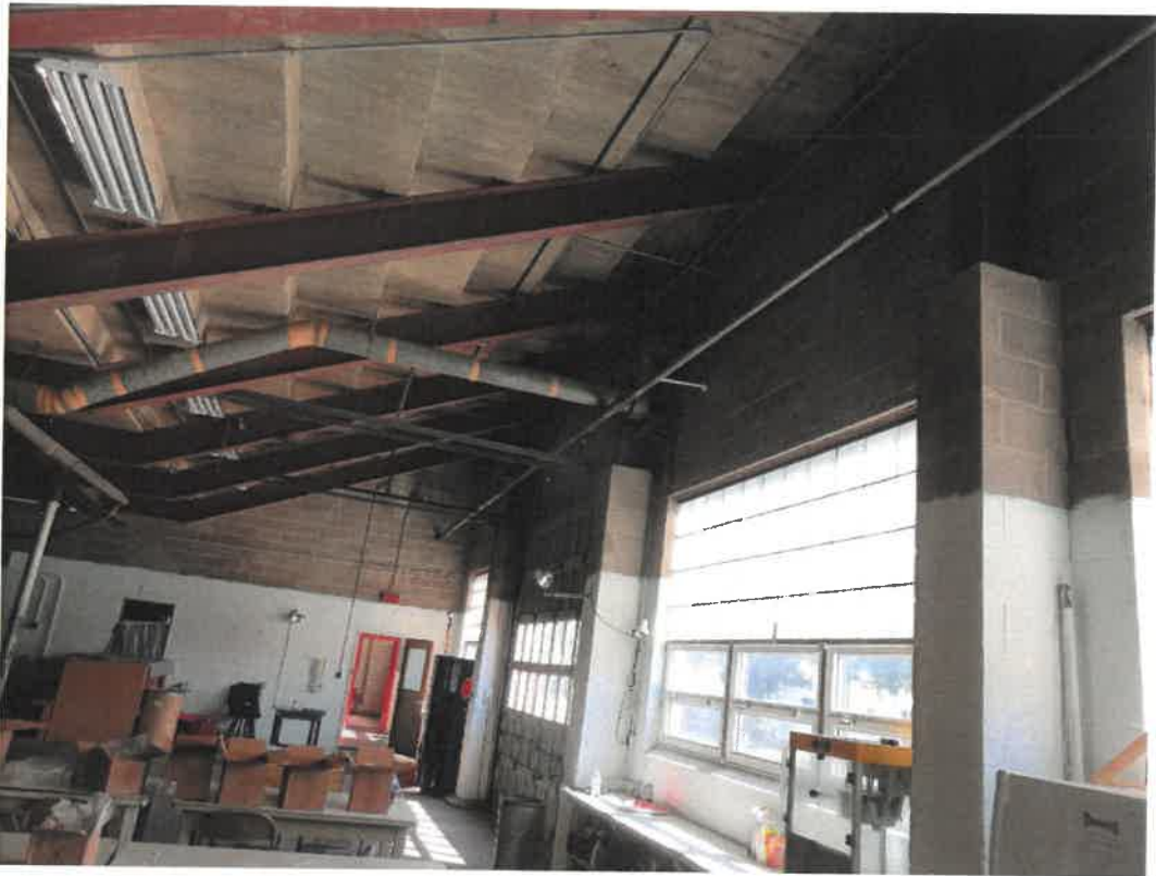
Photo 7 – Typical Steel and Cast-in-Place Concrete Construction beneath Bleachers
