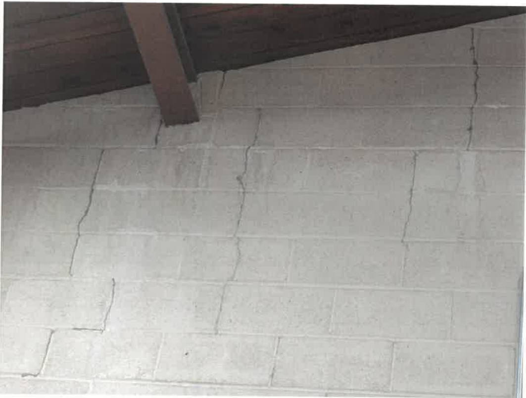
Photo 15 – Typical Cracks in CMU of Gymnasium with Indication of Past Water Infiltration into Cavity of Wall
