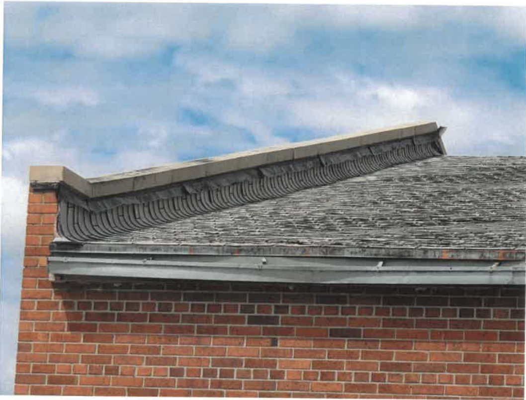
Photo 23 – Typical Aged Roof and Damaged Gutter
