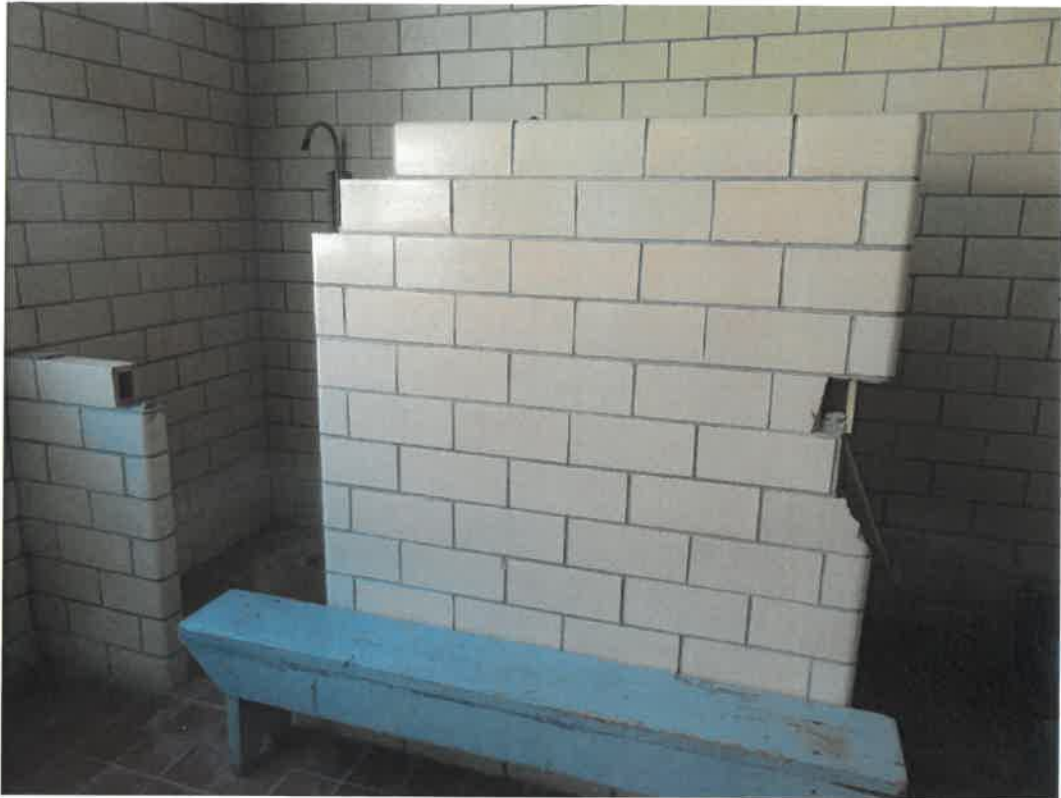
Photo 11 – Missing and Broken Tile Bricks in Restroom Partition Wall
