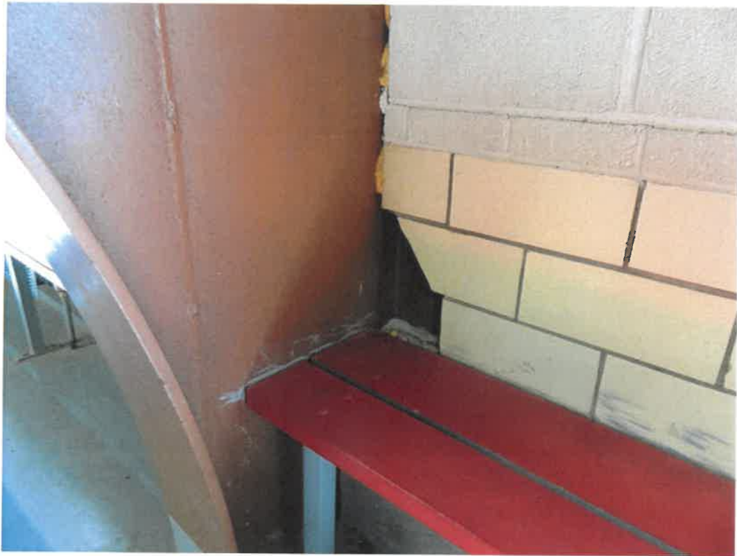
Photo 17 – Typical Missing and Broken Clay Tile Brick around Gymnasium Steel Columns at Top of Grandstand
