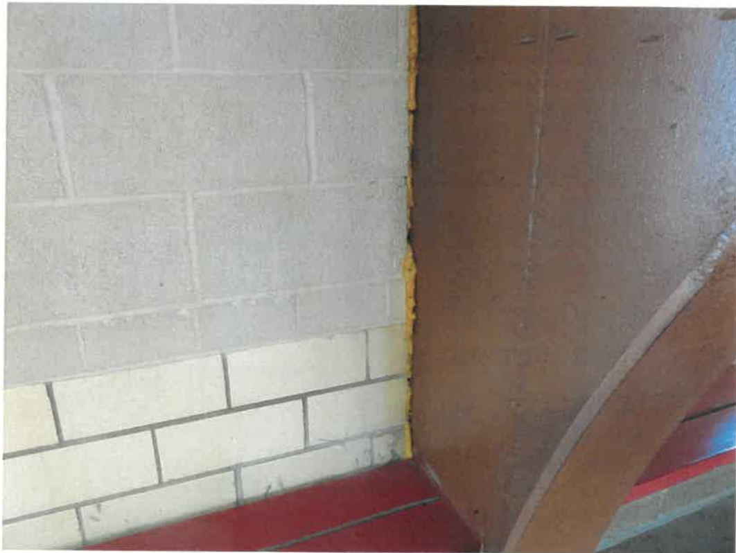
Photo 18 – Typical Foam Sealant Applied Around Gymnasium Steel Columns at Top of Grandstand
