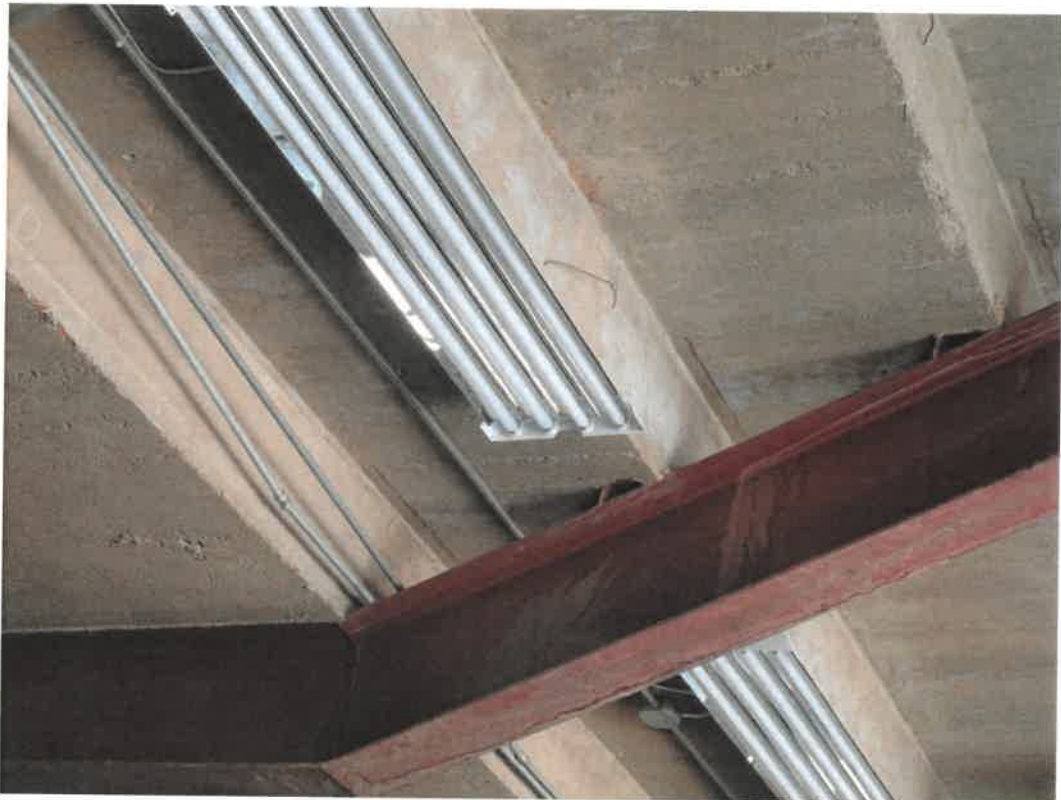
Photo 8 – Typical Steel and Cast-in-Place Concrete Construction beneath Bleachers
