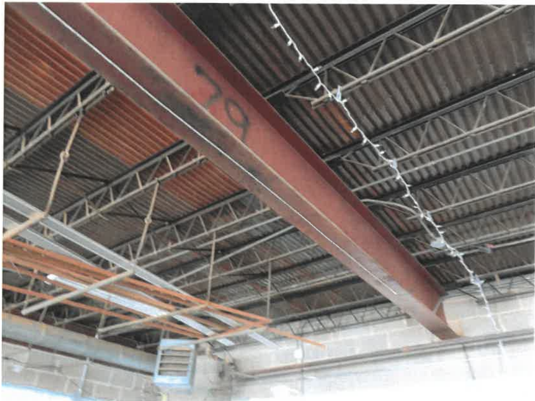
Photo 9 – Typical Steel Framing Construction beneath Stage
