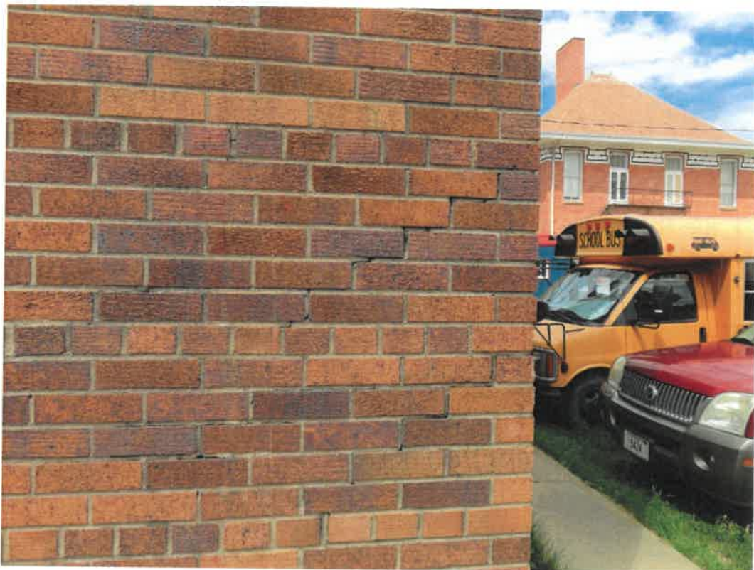
Photo 22 – Stair Stepped Crack in Brick at Northeast Corner
