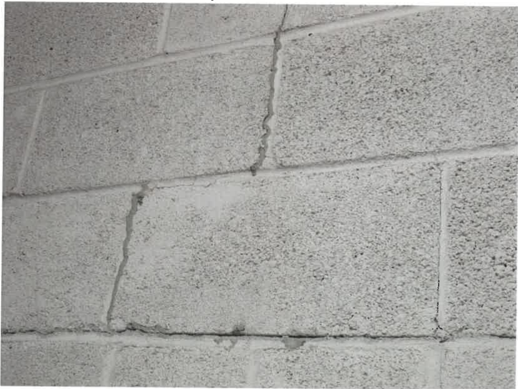
Photo 16 – Typical Aged Patching of Gymnasium CMU Wall
