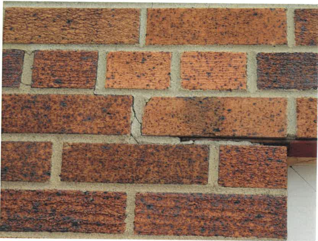
Photo 21 – Typical Missing and Cracked Mortar near Exterior Wall Opening
