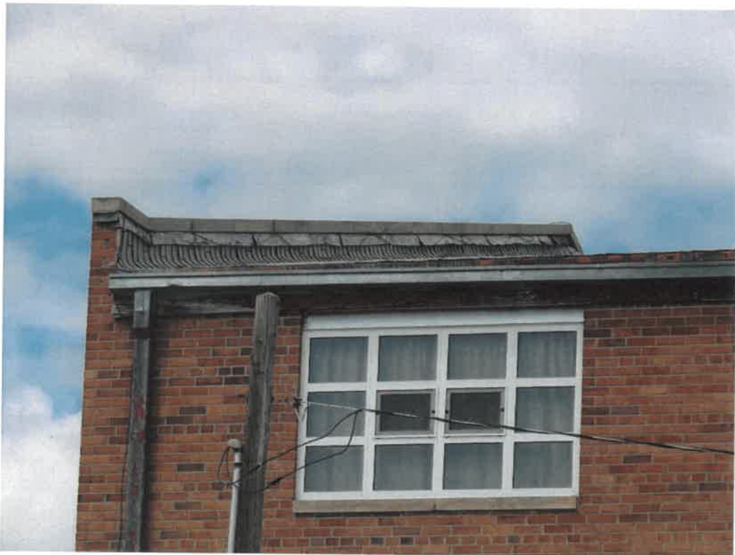
Photo 24 – Typical Aged Roof and Damaged Flashing
