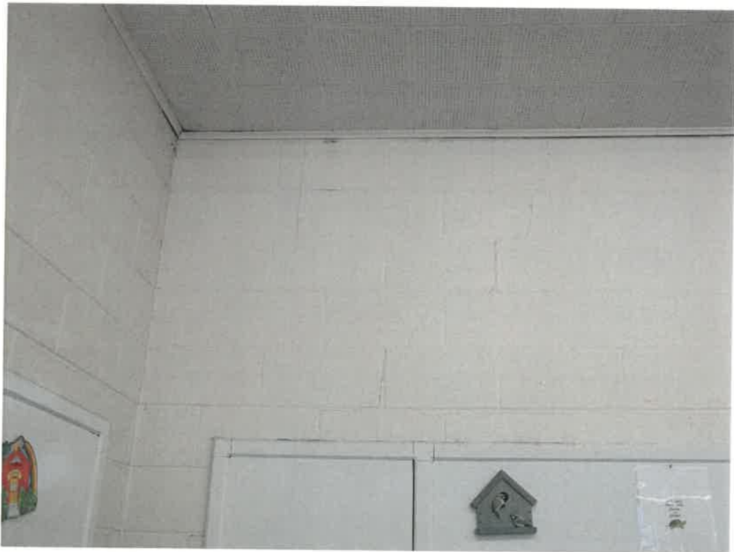
Photo 6 – Typical Crack in CMU Wall in Classrooms of First Floor
