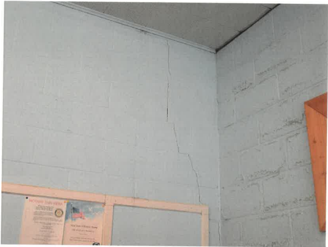
Photo 5 – Typical Crack in CMU Wall in Classrooms of First Floor
