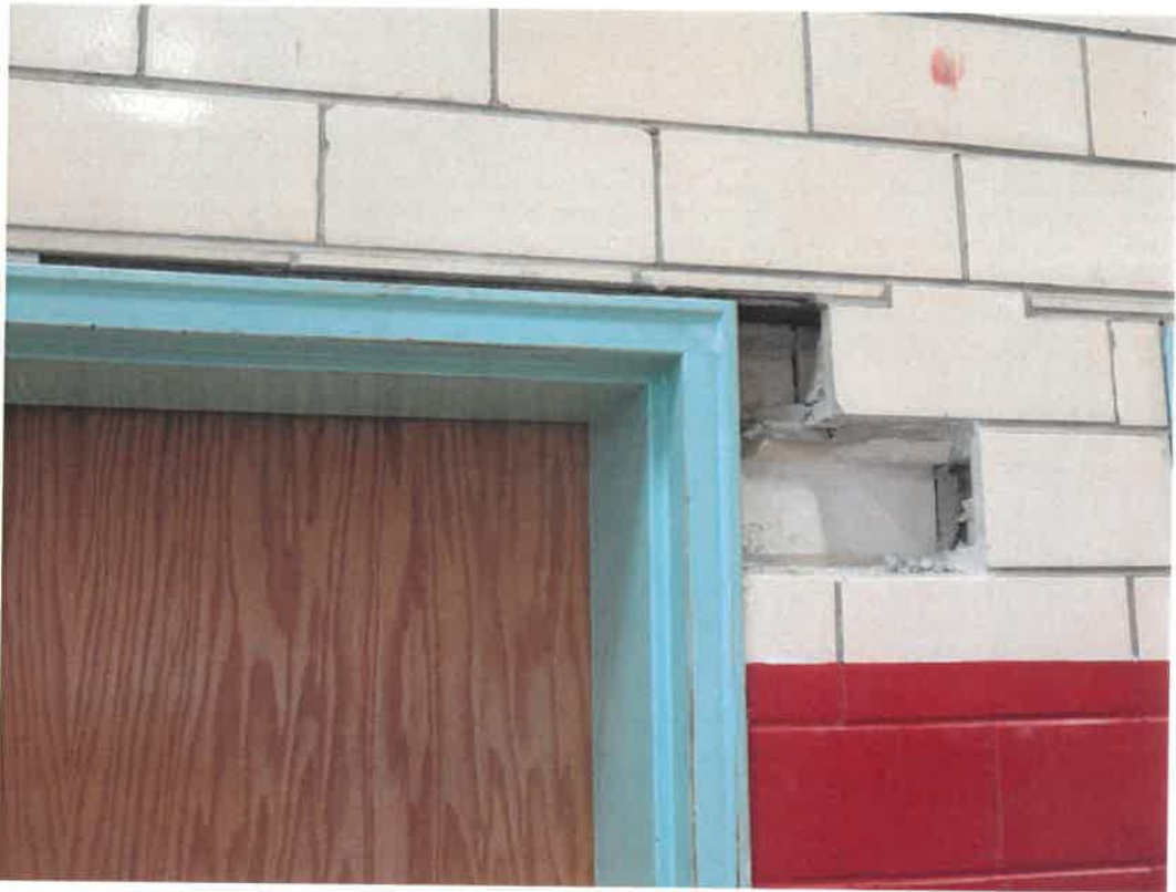
Photo 19 – Broken Clay Tile Brick at Walk Door in Gymnasium
