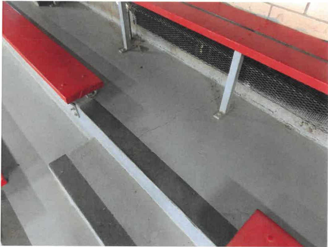
Photo 13 – Typical Hairline Cracks in Concrete Stands of Gymnasium
